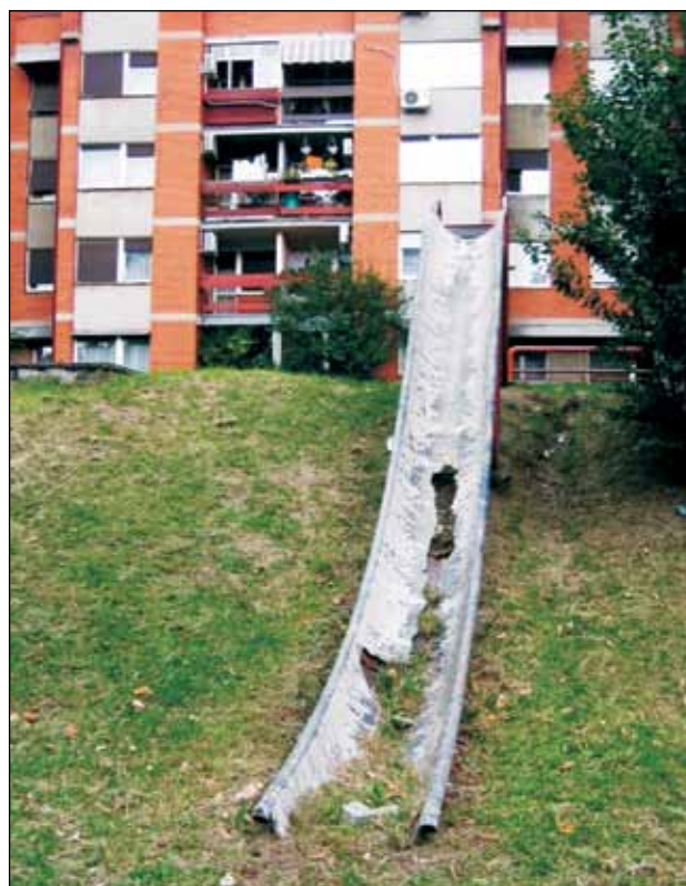
Figure 1. Ruined playground, which is dangerous for children's health
